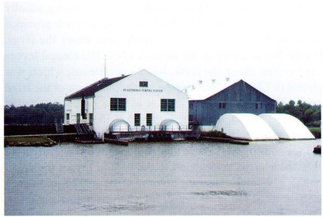
Figure 5 One of the city’s twenty-two large pumping stations.
