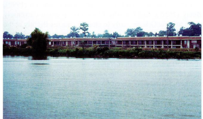
Figure 4 A motel complex behind a levee. The rooms on the first floor are below sea level.
